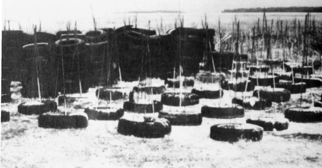
Figure 10.—Eight-tire units are quickly constructed by assembly-line techniques.
